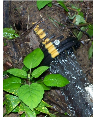
Figure 1: Water drains from the main outlet of a field tiled using Intellislope
